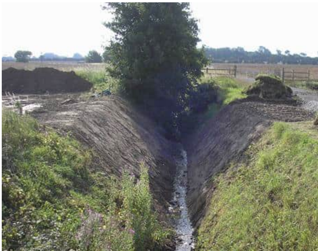
Plate 10. Example of a reinstated watercourse immediately following open-cut cable installation
